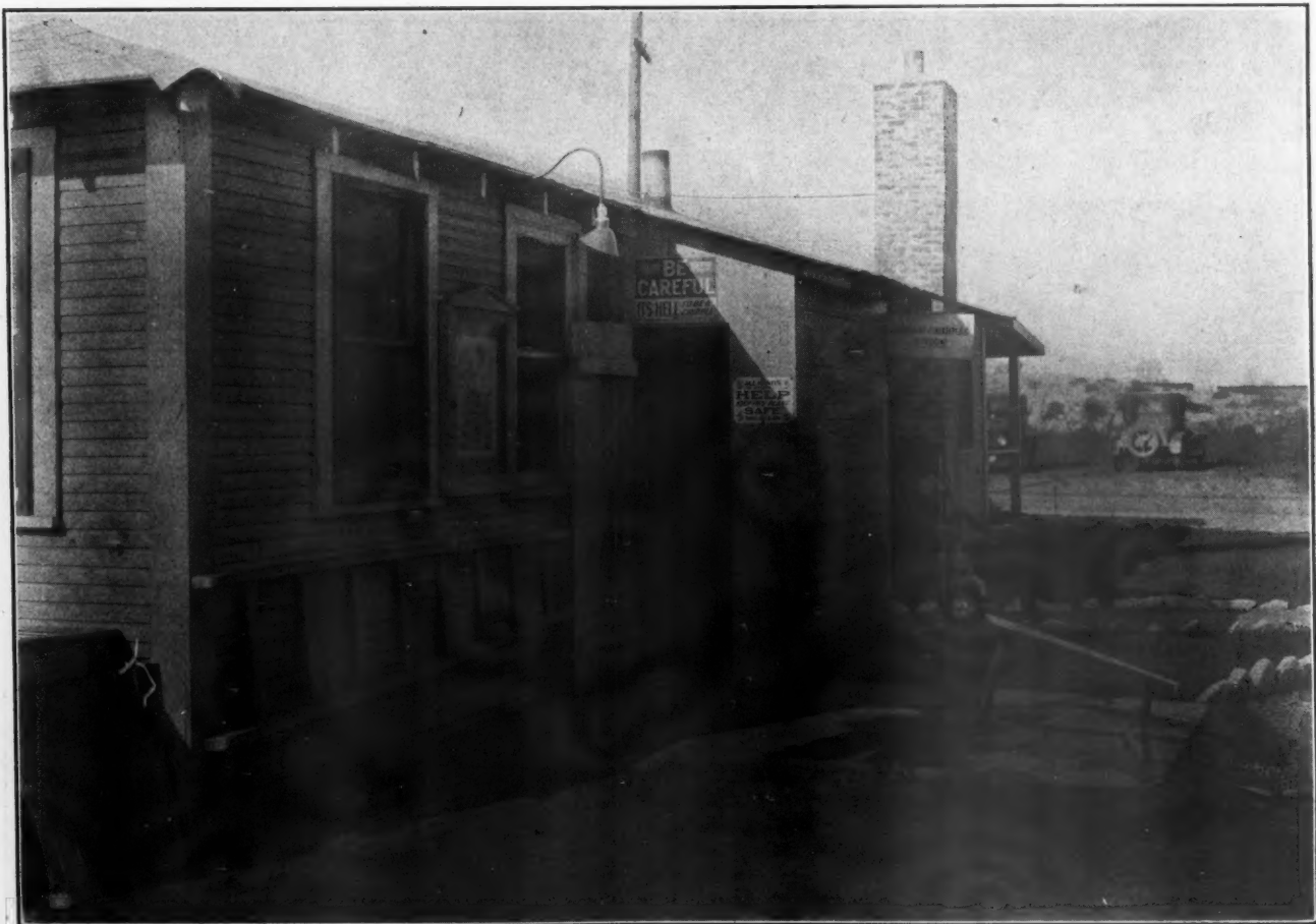
Keep Plant Clean—Painted and Tidy. Note Safety Sign Placed at a Psychological Place—The Employment Office.
